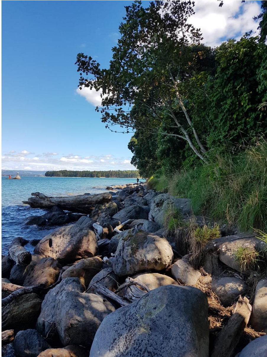
Figure 8: General view of the area of terrace 18 (at right of photo), within the construction footprint of the revetment and new base track section (photo credit, InSitu Heritage Ltd, March 2018).
